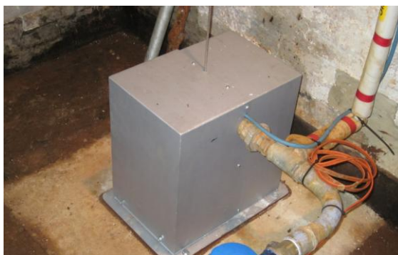
Headworks after improvement with protective cover.
