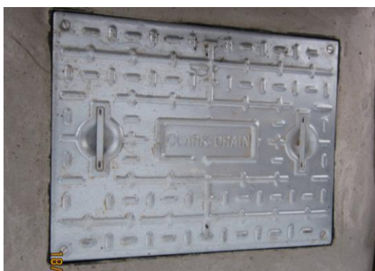
Reservoir hatch after improvement with additional fixed cover.
