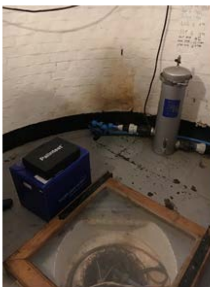
Figure 9: Borehole headworks
