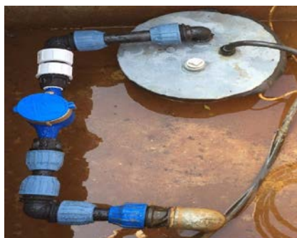
Figure 27: Poorly constructed headworks on source
