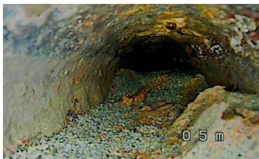
Figure 26: Sediment in pipework
