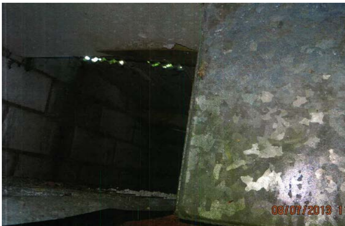
Figure 19: Storage tank with holes in roof
