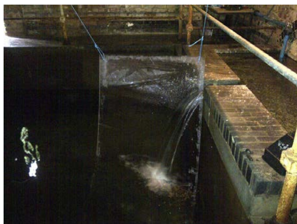
Figure 14a: Rudimentary arrangement for chlorine mixing (perspex sheet)
