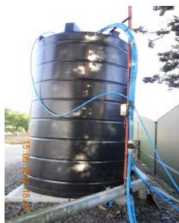
Figure 21: Tanks in which mains water and borehole water were blended and stored
