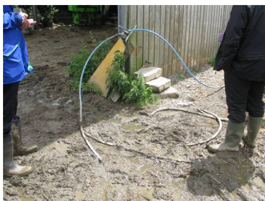
Figure 9: Contraventions of fittings regulations in relation to pipes and animal troughs
