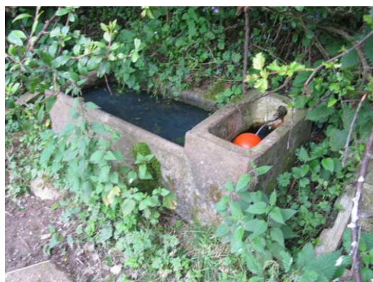
Figure 9: Contraventions of fittings regulations in relation to pipes and animal troughs
