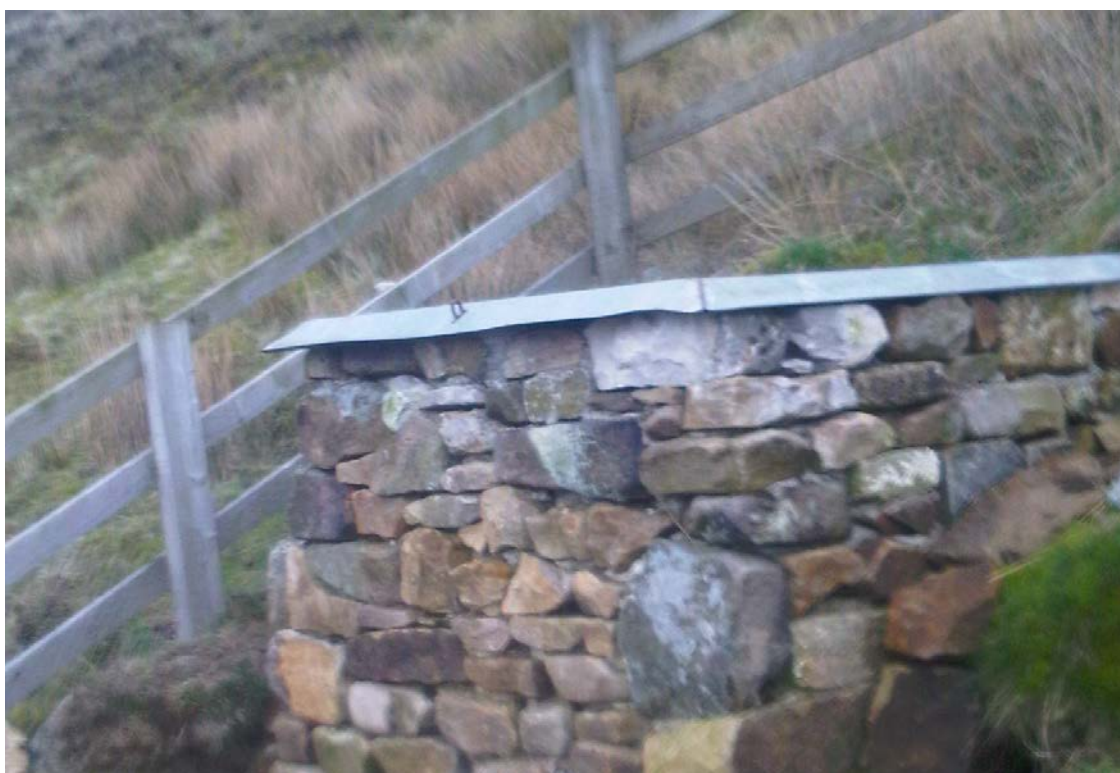
Figure 12: Spring chamber located on a steep slope, surrounded by fencing (0.5 m from the chamber) and boggy land and swallow holes
