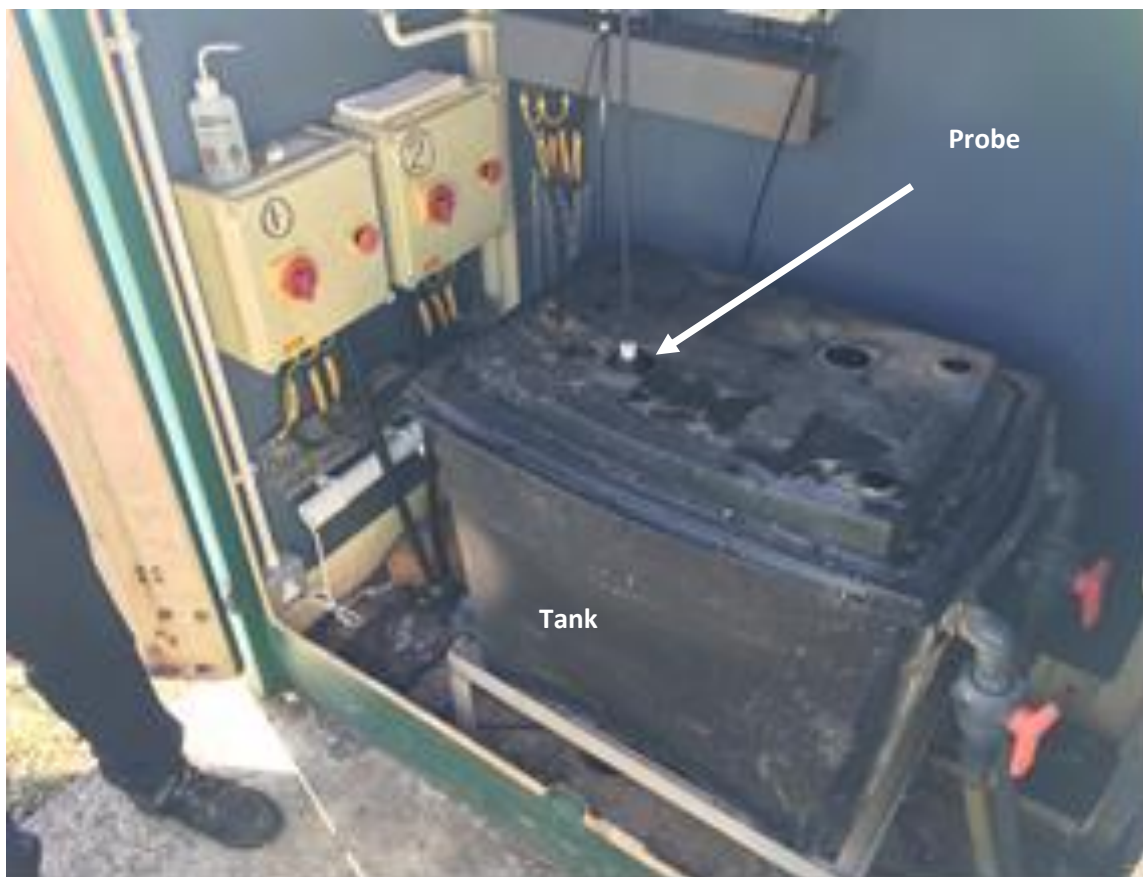
Figure 3: Sample tank for supernatant turbidity monitor at Iver works
