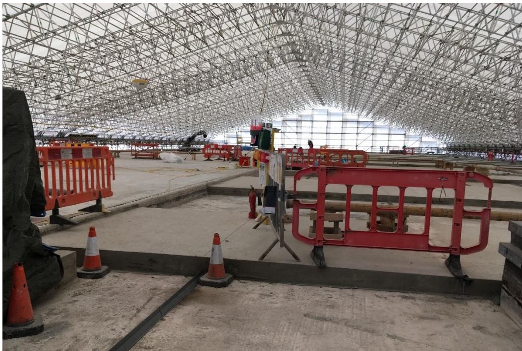
Figure 7: Protective cover over the contact tank at Severn Trent's Strensham works
