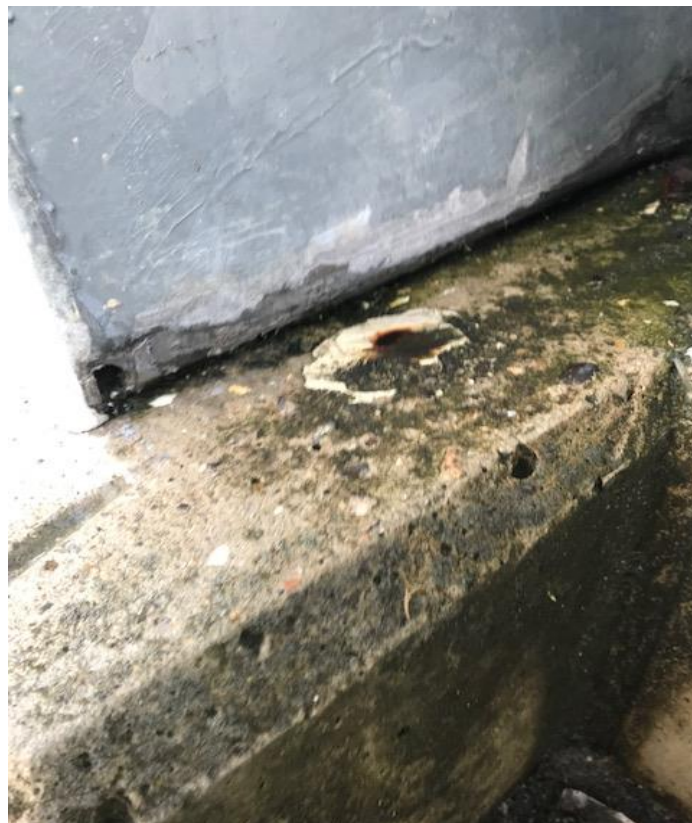
Figure 5: Missing hatch seal on Chingford Contact Tank
