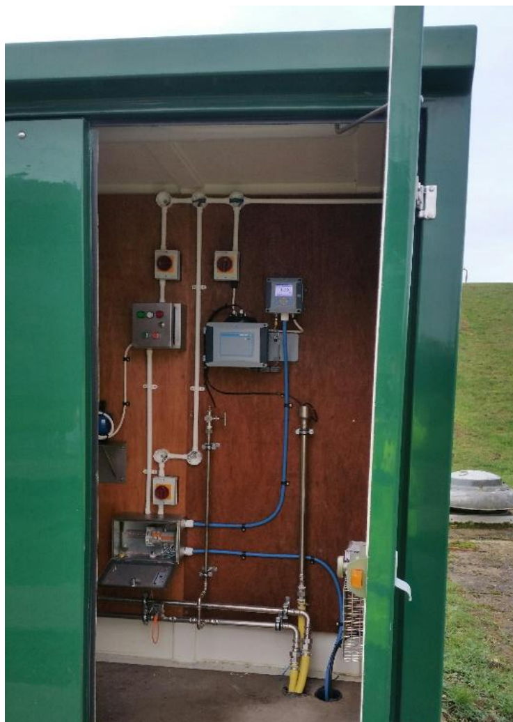
Figure 4: New supernatant turbidity kiosk at Iver works
