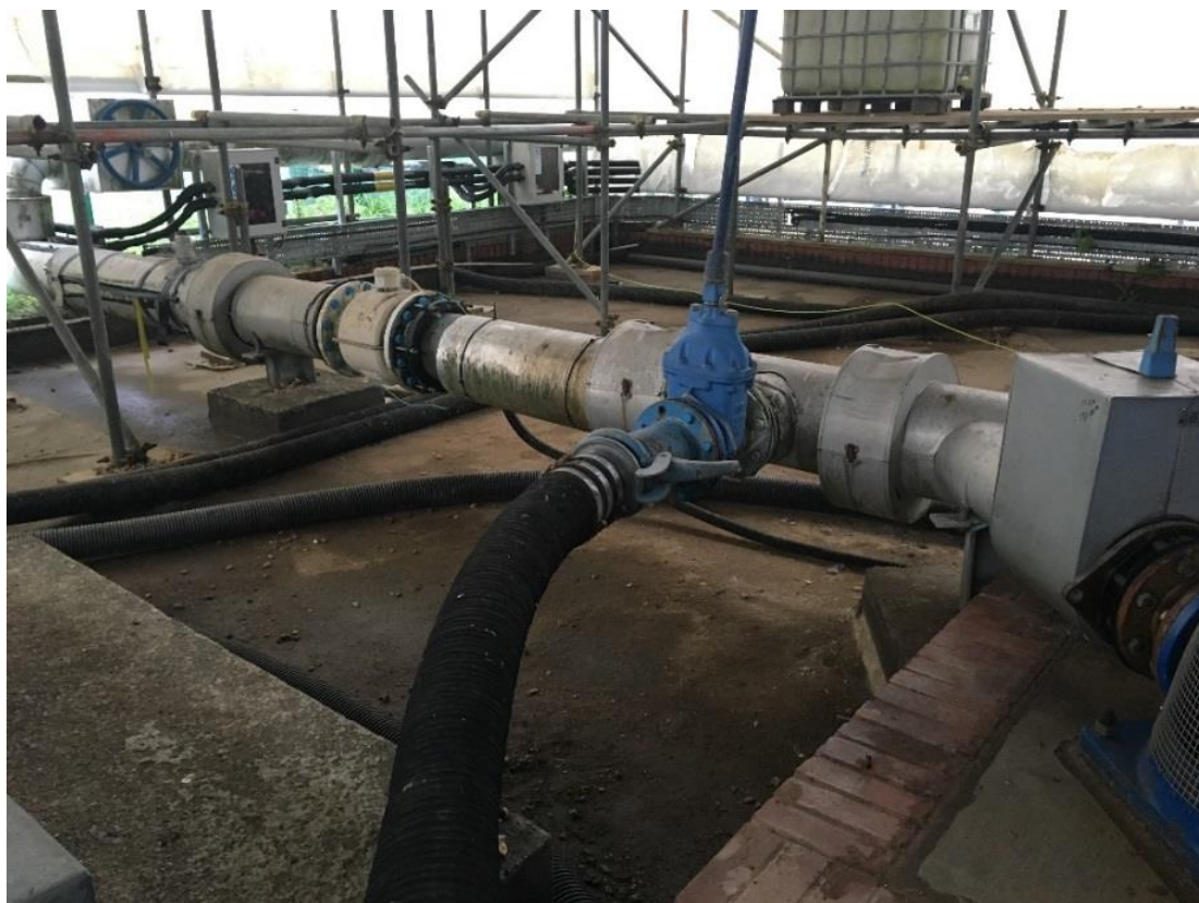
Figure 11: Temporary hose connected to treated water main at Sandown works
