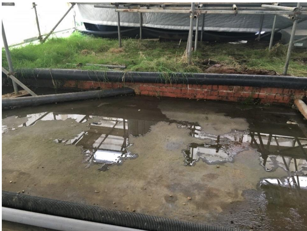
Figure 6: Ongoing run off of surface water onto Sandown's contact tank roof
