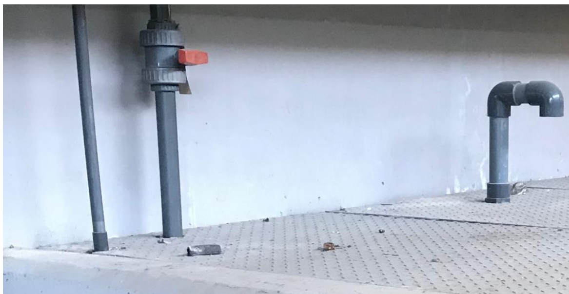
Figure 8: Debris and poor fitting plates above the filter outlet channel at Iver works
