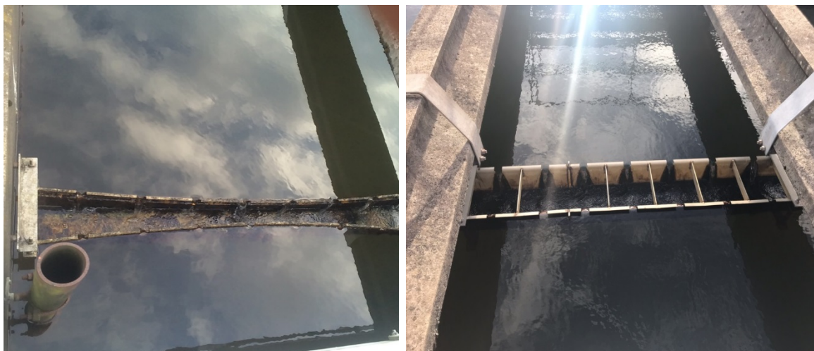
Figure 1: Warped GRP Launderers (left), Replaced with Steel at Sluvad works.
