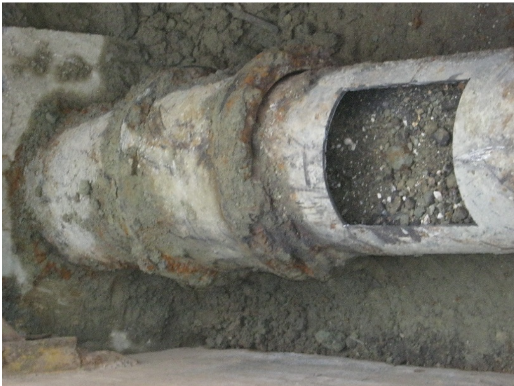
Figure 7: Soil ingress in the inlet pipe of Cooks Castle service reservoir.
