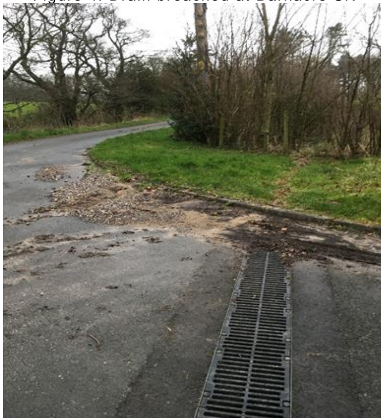
Figure 4: Drain breached at Barnacre SR
