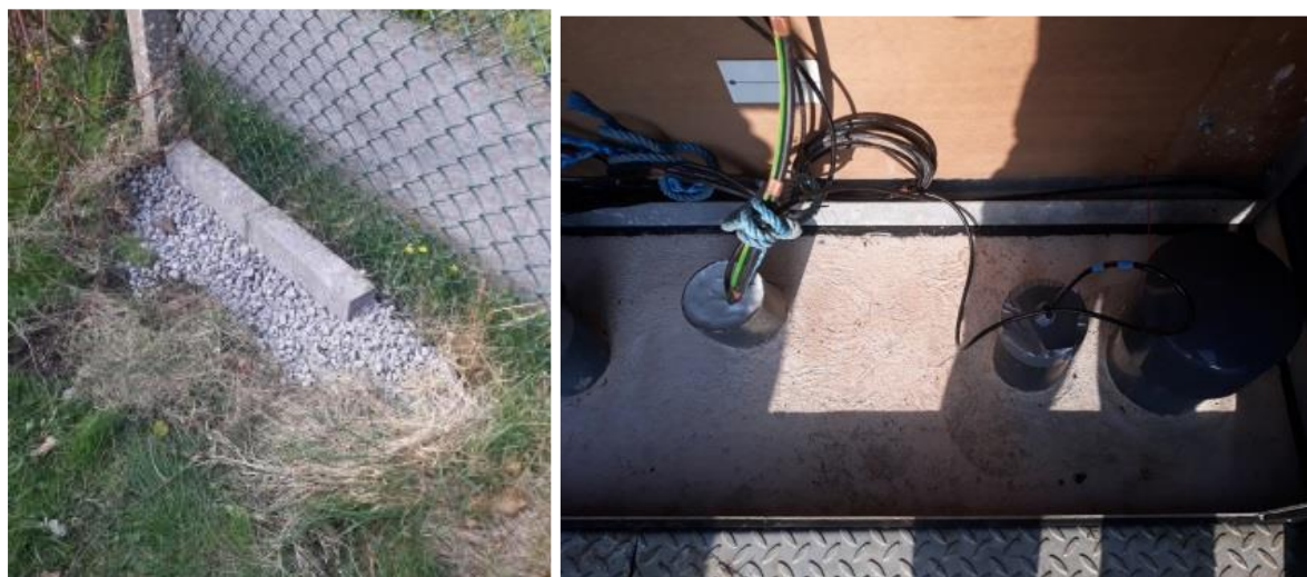
Figure 5: Fence repairs and sealed ducts among measures to address vermin risks at Cheddar works
