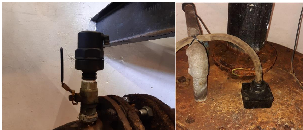
Figure 6: Air valve replaced, and gland fixed following the audit at Ford works
