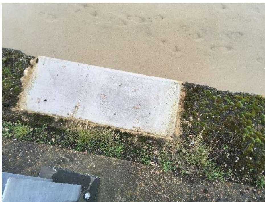
Figure 2: Repaired coping stone among excessive vegetation at Ashford Common works
