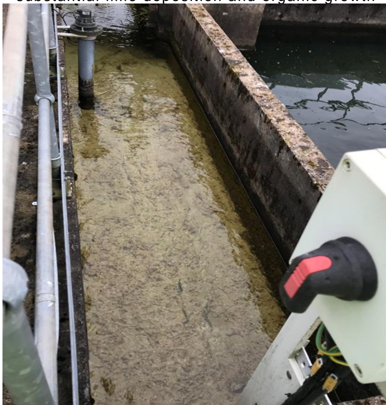
Figure 3: Fontburn rapid gravity filter inlet channel showing substantial lime deposition and organic growth
