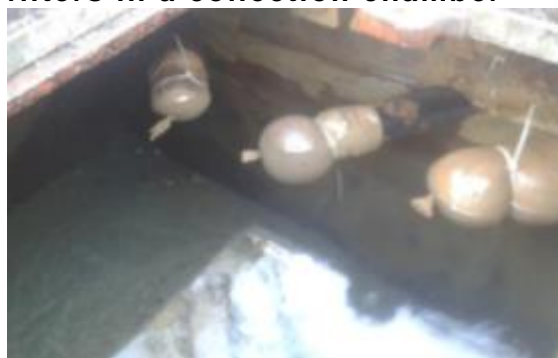
Figure 26: Tights being used as filters in a collection chamber
