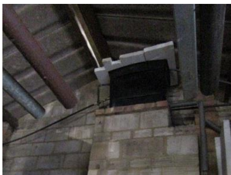
Figure 23: Header tank with overlaid polystyrene strips as a cover
