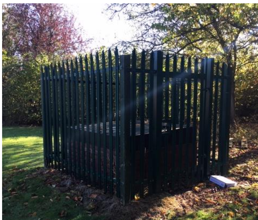
Figure 30: Robust source protection on a private supply to a hospital
