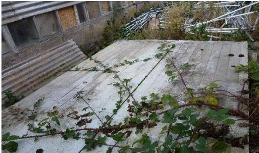
Figure 21 : Vegetation covering poorly constructed well cover
