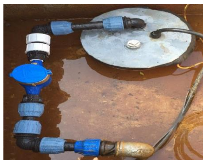
Figure 28: Poorly constructed headworks on source
