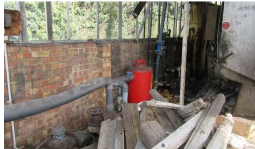
Figure 22: Supply pipework in an inadequate and unacceptable environment
