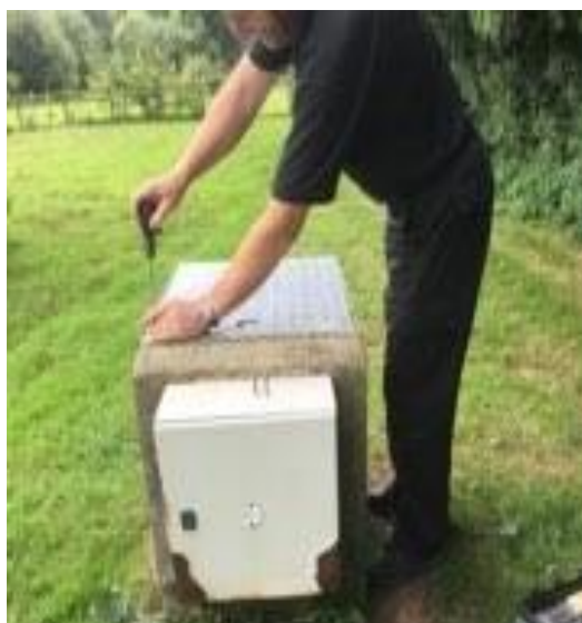
Figure11: Example of raised chamber to protect well head from ingress
