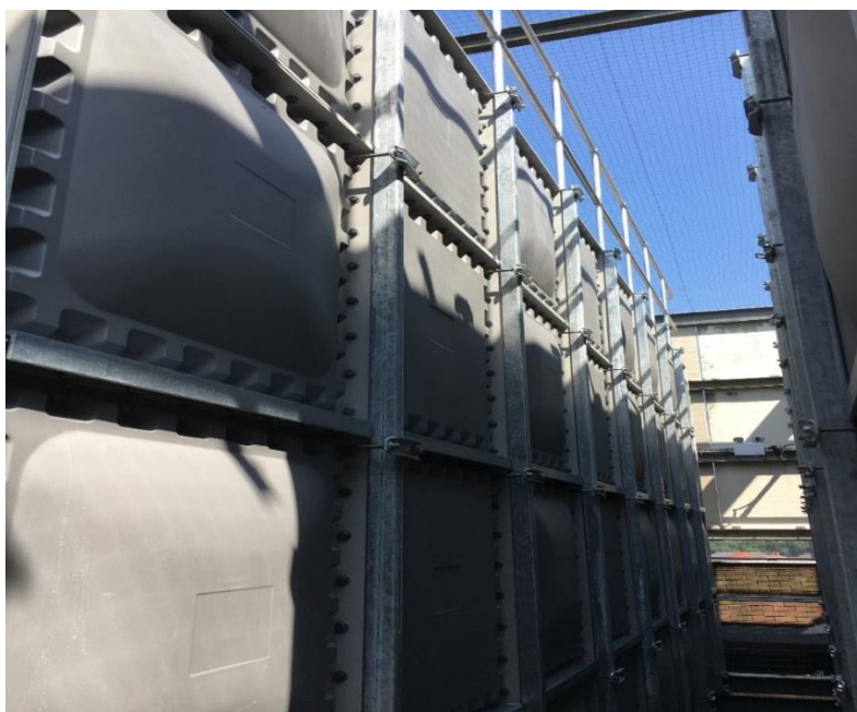
Figure12: Insulated and protected treated water storage tanks
