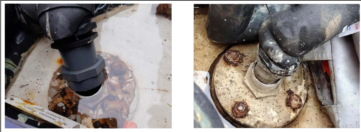
Figure 1: Unsealed dosing lines at Coppermills works
